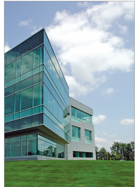
Mindray North America Headquarters 800 MacArthur Boulevard Mahwah, New Jersey 07430 Tel: (201) 995-8000
